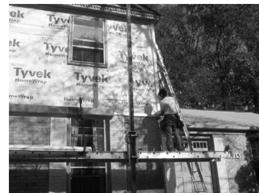
Best Siding Contractors at work on one of the houses
