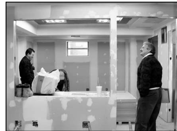
(Above) Stevens Brown (right), a senior planner with Montgomery County's Department of Housing and Community Affairs and Mario Martinez (left), a program manager's assistant with CASA, inspect progress in what will be the Center's computer lab.
