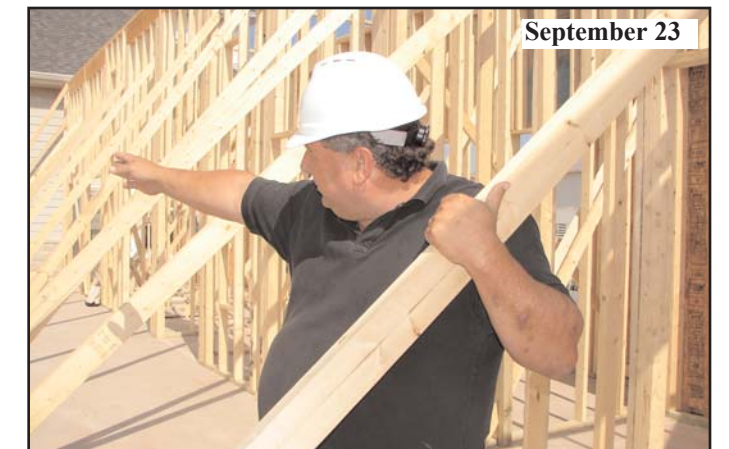
Winchester's Ron Keefer onsite and in charge.
