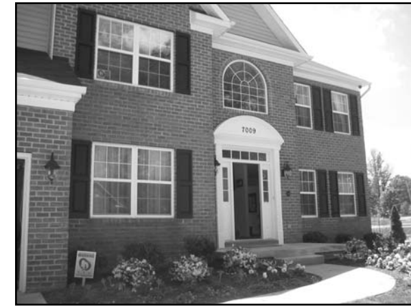
The new four bedroom house is located in Clinton, MD.
