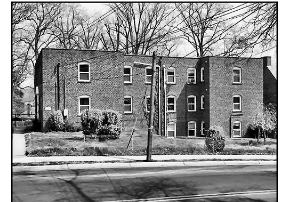
Located at Dale Drive, the property is a three-story brick building containing 10 small one-bedroom units
