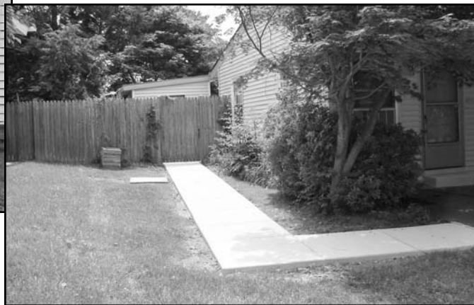
After: Brand new sidewalk.
